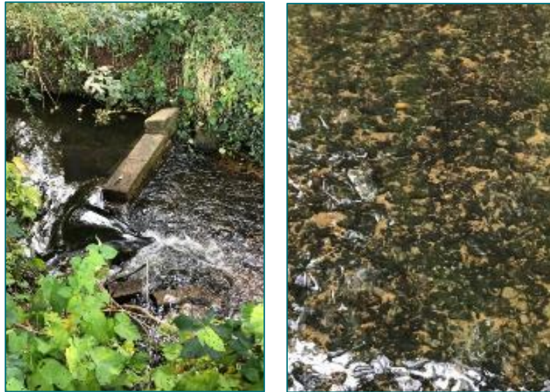
Plate 20.3.15: Weir and bed armouring along the Swannington Beck.
