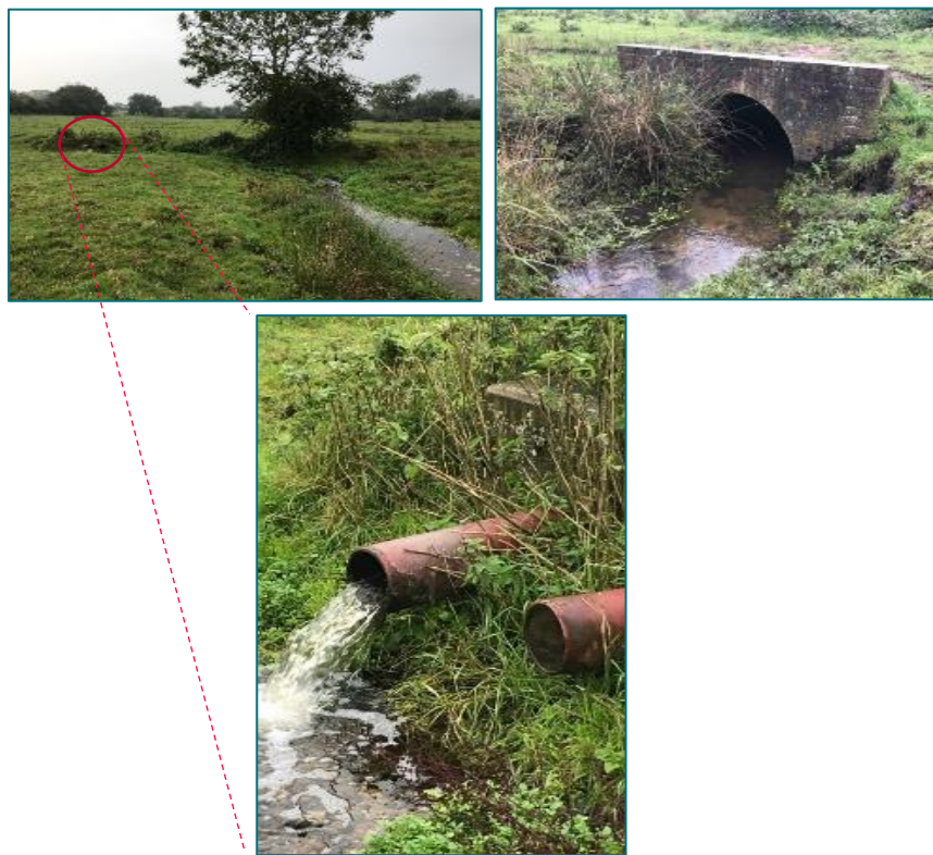
Plate 20.3.39: Outfall pipe and small culvert.
